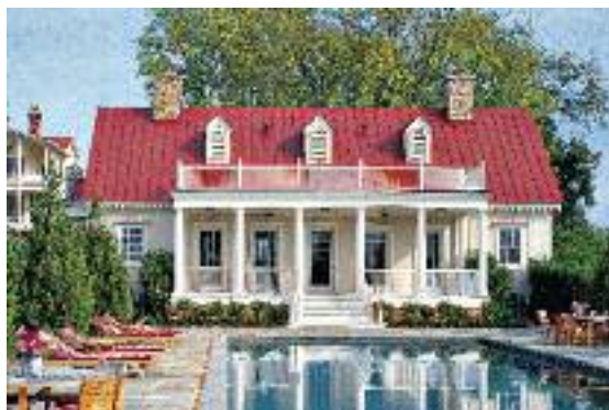
This pool house on a Virginia farm reflects the local vernacular in its raised-seam, red-painted tern roof, and its five-bay porch echoes that of the main house.
